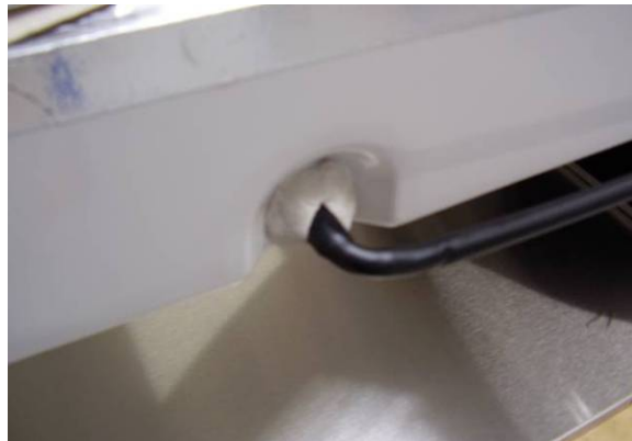
Figure 17: Drain pipe and putty
